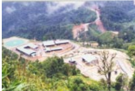
The heliport at this Total pipeline station was built with forced labor. Photo:ERI
